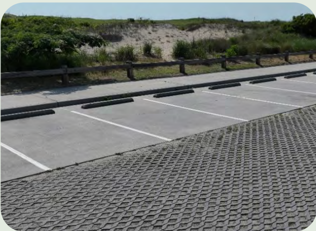
Monolithic concrete parking adjacent to cellular grid pavers allowing for more parking accessible to all users at Little Island Park.
