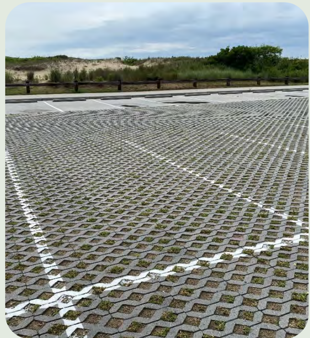
Cellular grid pavers installed at Little Island Park in Sandbridge. Note the grass growing in the cells - this will help reduce runoff even further.
