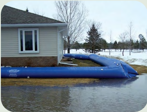
A water filled temporary barrier surrounding a house, in place before flood waters rise. Image courtesy of FEMA
