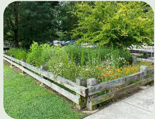
Bio-retention bed with rain garden at Redwing Park designed to support dry ground plants.
