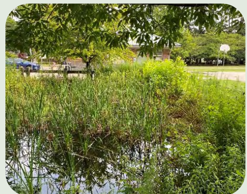
Bio-retention bed with rain garden at Redwing Park designed to support marsh plants.
