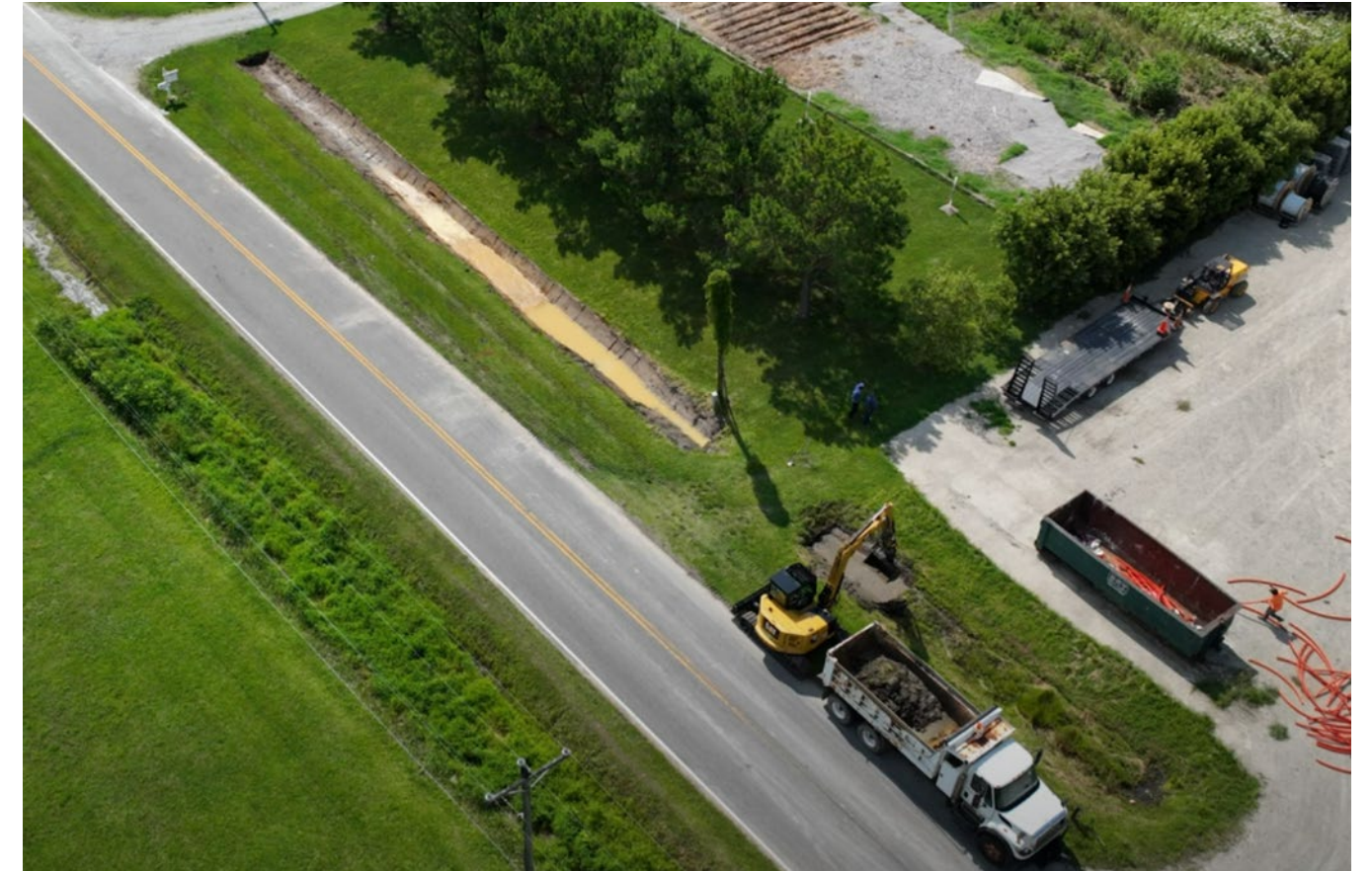
Public Works Operations removing sediment and debris from a roadside ditch and placing it into a dump truck
