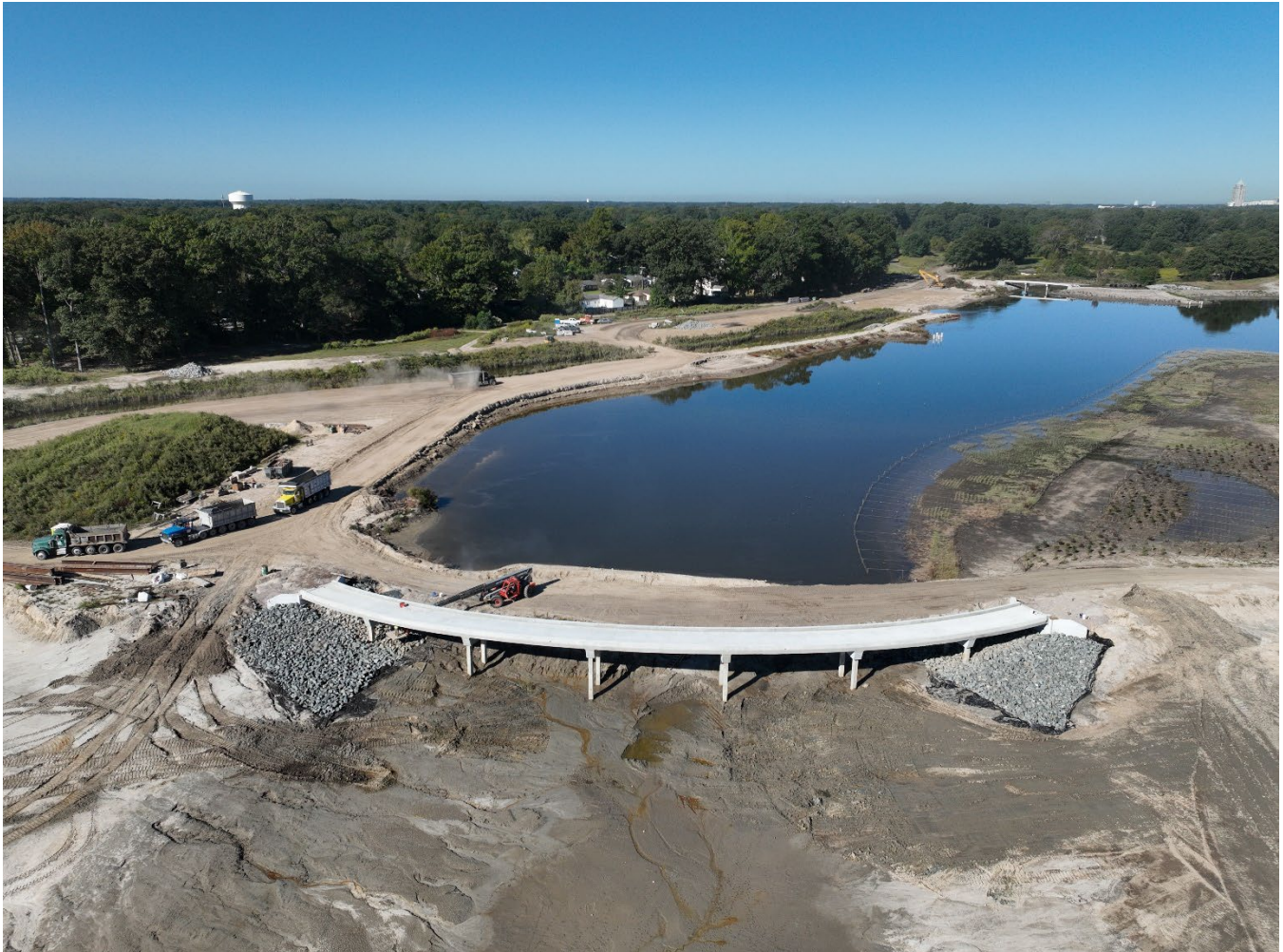
Bow Creek Stormwater Park showing Pedestrian Walkway #2 in the foreground with a large expansive impoundment in the background. Note the new plantings on the right side of the image.
