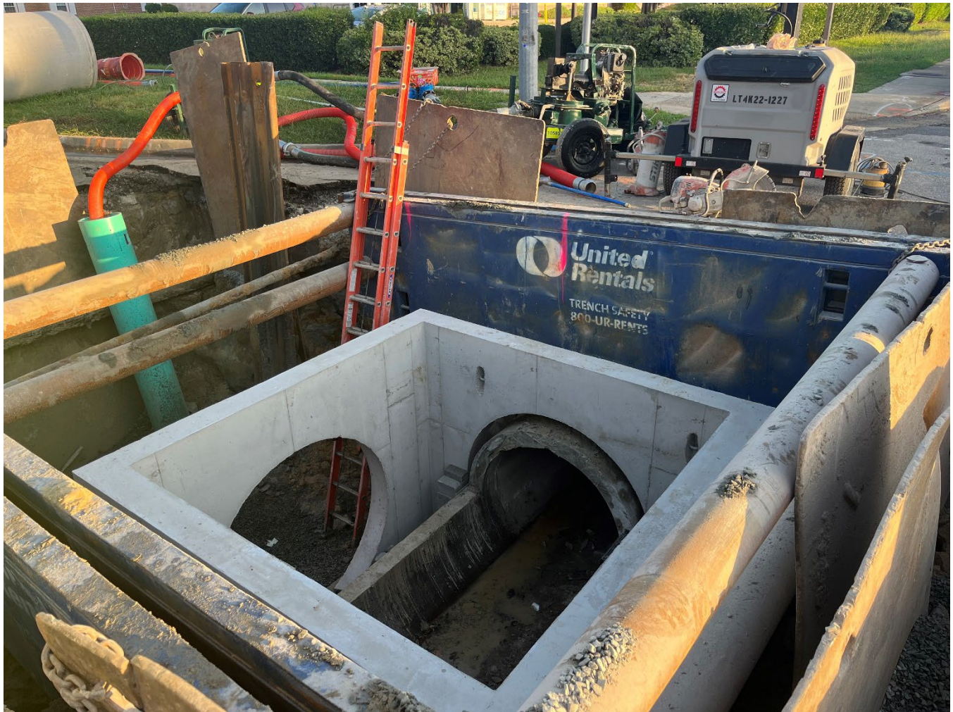
Installing a doghouse junction box over an existing storm pipe for the S. Plaza Trail and Presential Boulevard Drainage Improvement Project at the intersection of Rosemont Rd and S. Plaza Trail.
