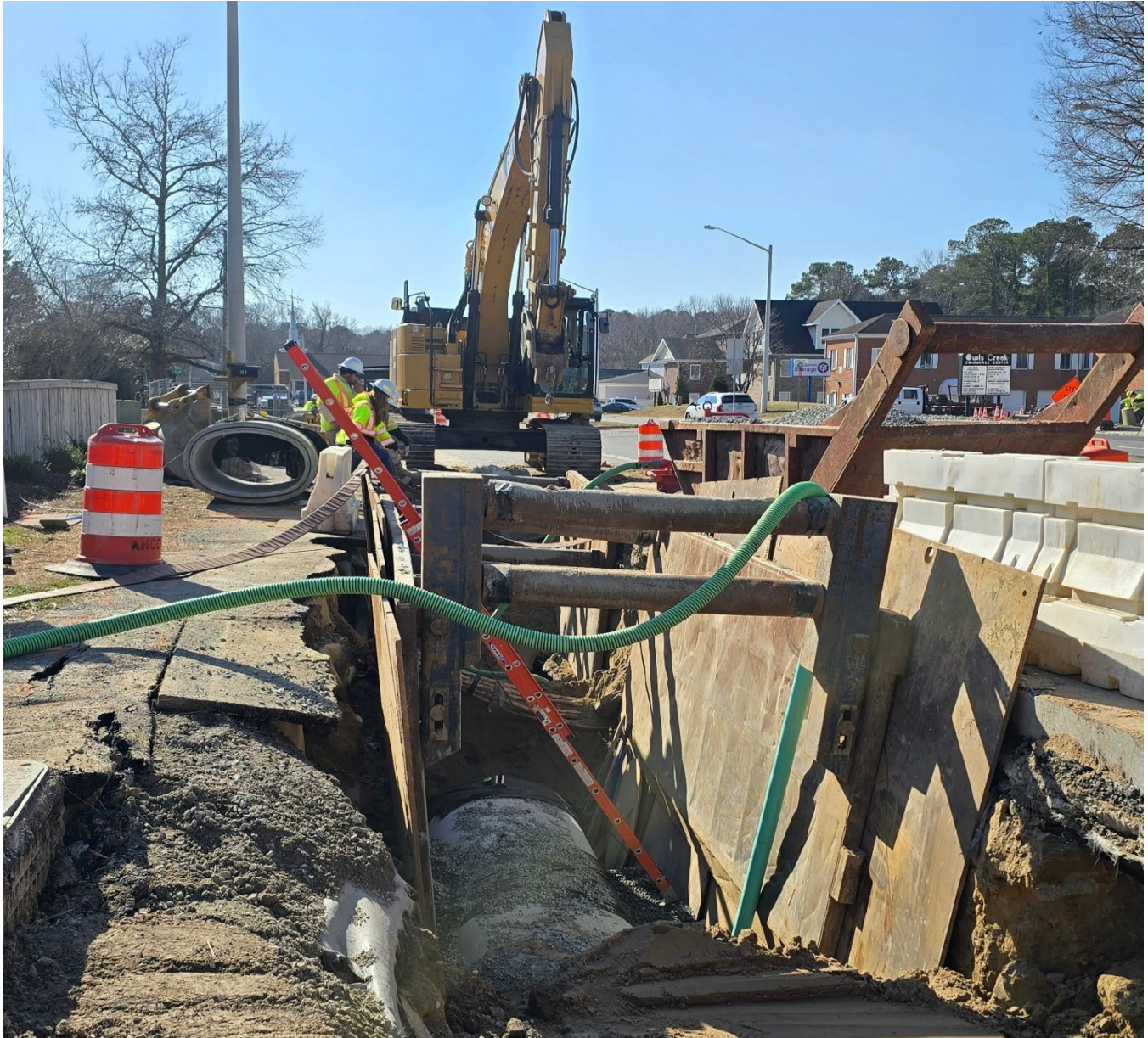
Seatack Neighborhood Improvements: Installation of 45in x 29in elliptical storm pipe on Birdneck Road (northbound) near the intersection of Burford Ave.
