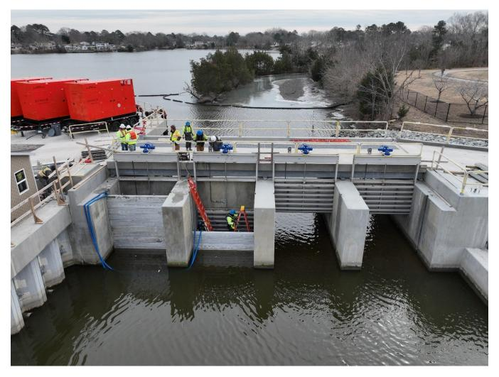
Working on the finishing touches at the Windsor Woods Tide Gate. Note the stop logs in place to assist with maintenance on one of the four gates and the temporary pumps in orange.
