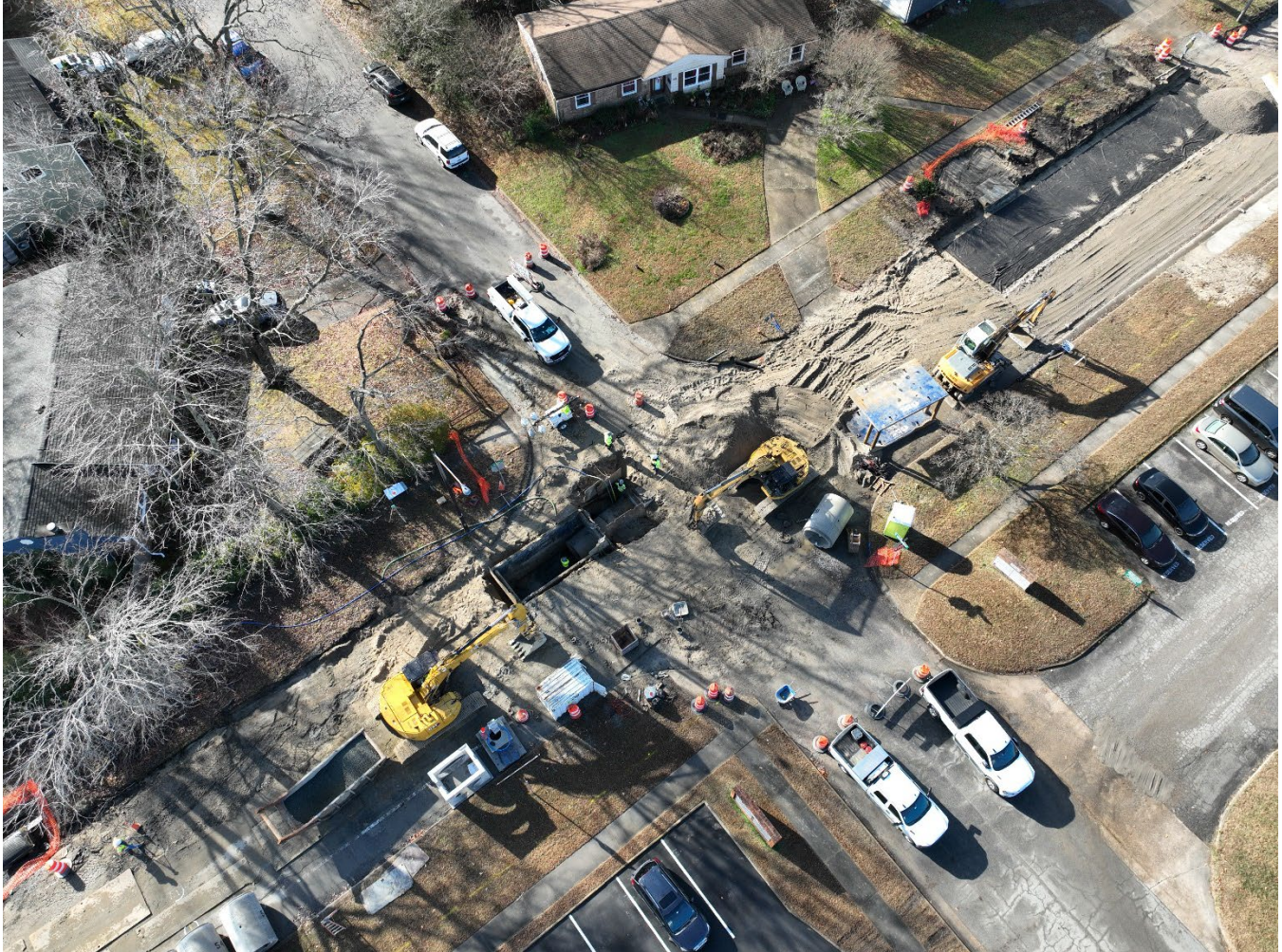
South Plaza Trail and Donna Wood Drive intersection installing 54 inch diameter stormwater pipe.
