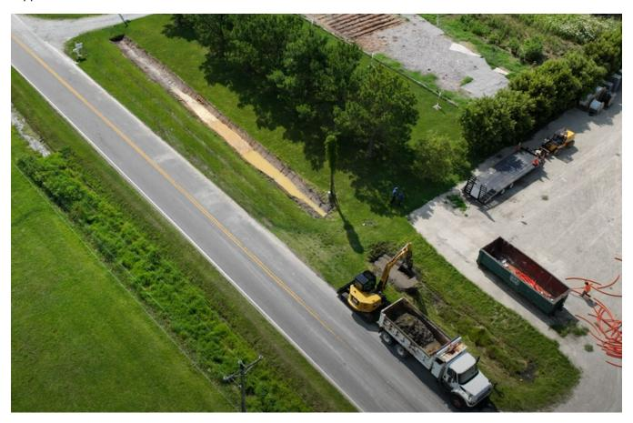
Public Works Operations removing sediment and debris from a roadside ditch and placing it into a dump truck.
