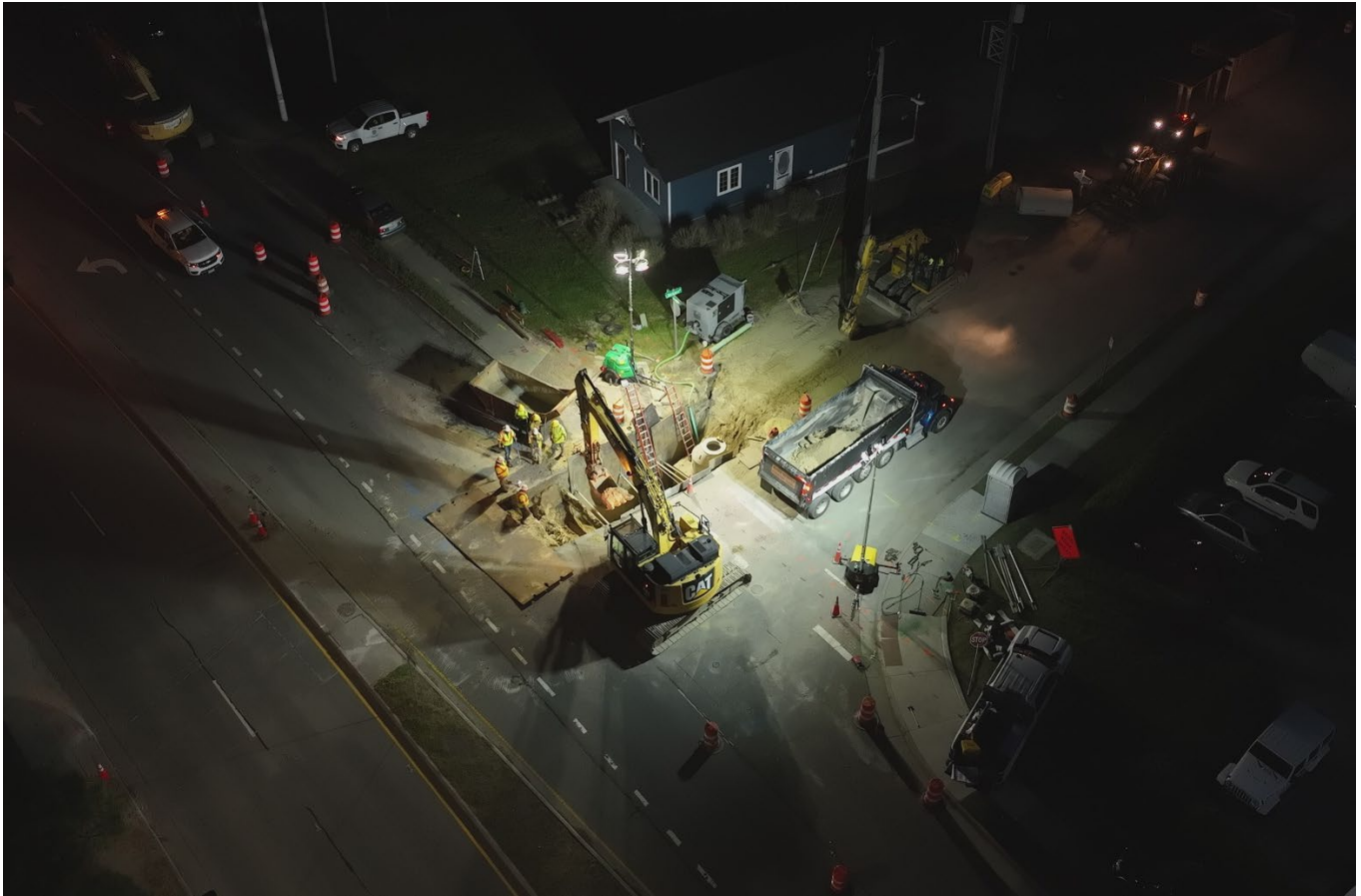
Seatack Drainage Improvements – Night work to install a 53in x 34in horizontal elliptical storm pipe across Birdneck Road.
