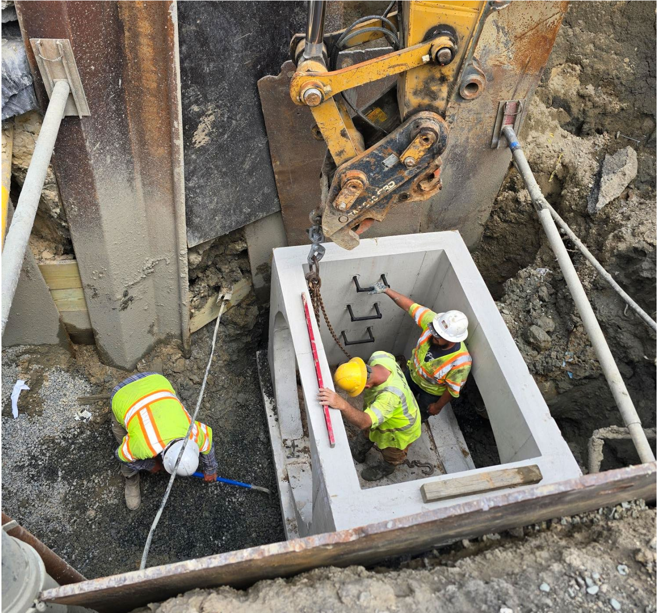
A storm structure being set at the Seatack Drainage Improvement project.
