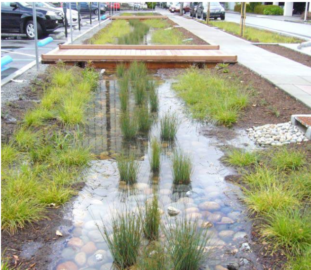
FIG. 4.2.27 RAIN GARDEN IN BAY AREA GREENBELT San Francisco, California
