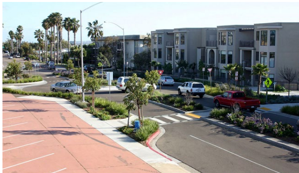
FIG. 4.2.12 MID-BLOCK CURB EXTENSION
