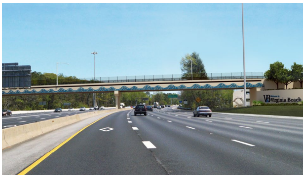
FIG. 4.4.10 WITCHDUCK ROAD FLYOVER Virginia Beach, Virginia
