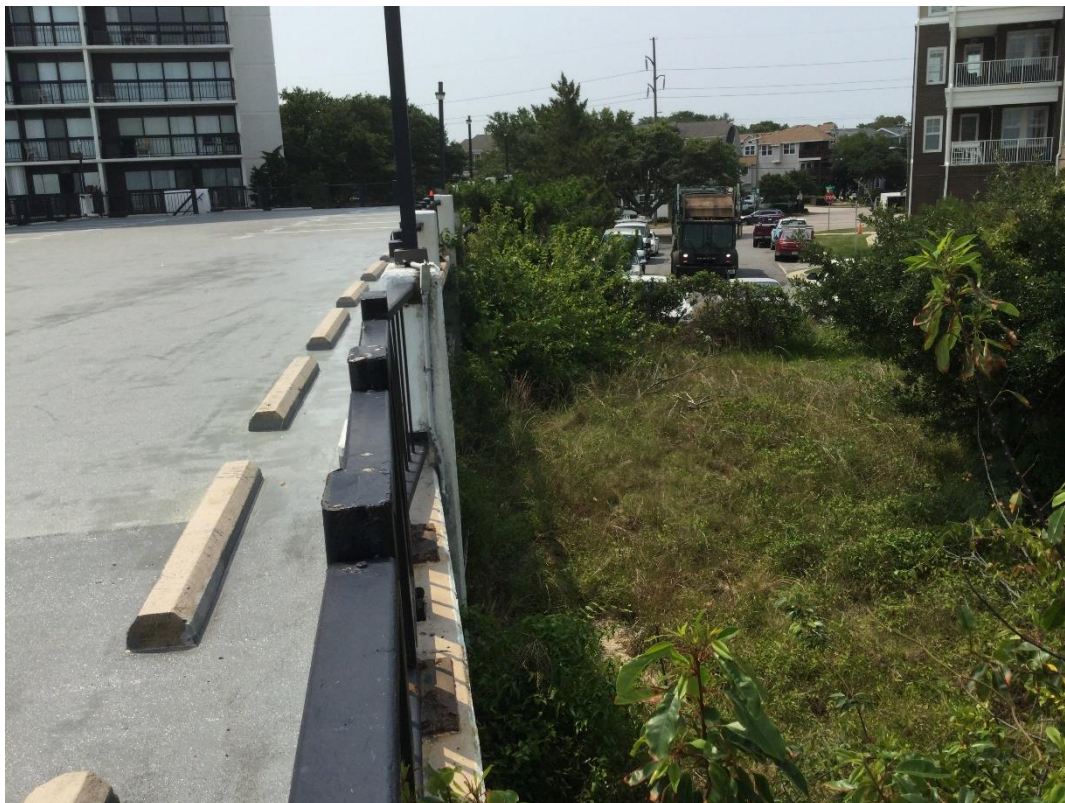
Photo 4: View of sand dune encroachment into first level of parking garage taken from second level of parking garage at Chesapeake House on the Bay
