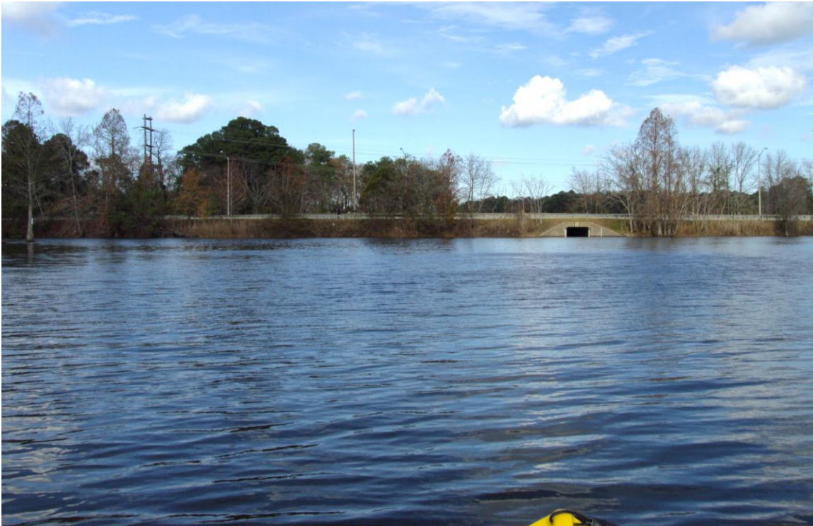
Photo 22. Weir Between Lake Smith and Little Creek Reservoir
