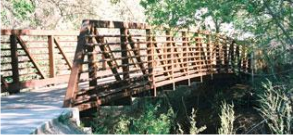
Photo 41. Sample Bridge Photo - Weathering Steel Superstructure & Wood Deck
