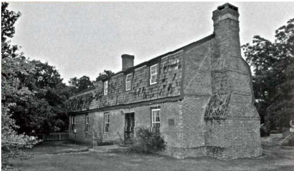
Photo 25. Weblin House Historic Photo
