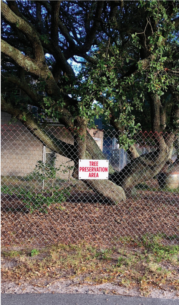
Tree Preservation Area on a Construction Site, Virginia Beach, VA
