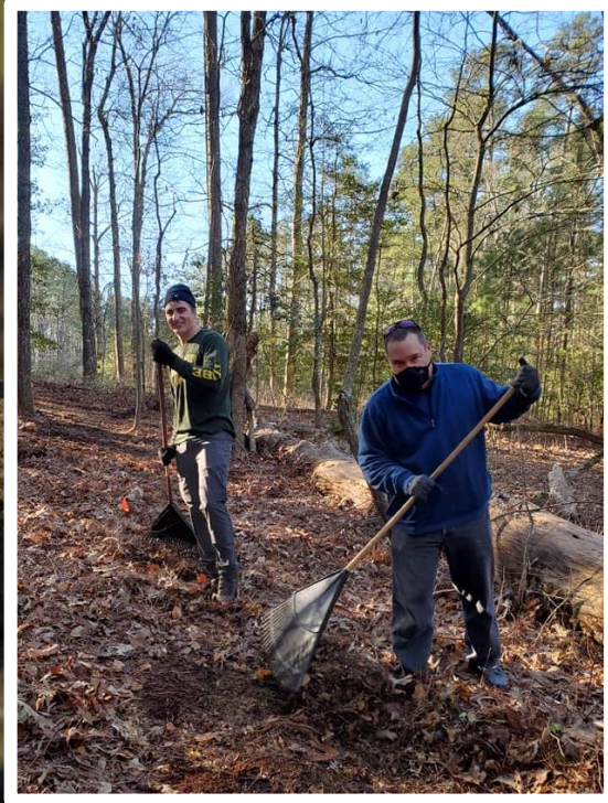
Trail design & construction
