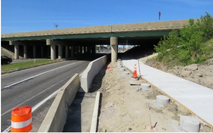
Witchduck embankment path under construction
