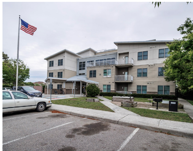
Cedar Grove Apartments
