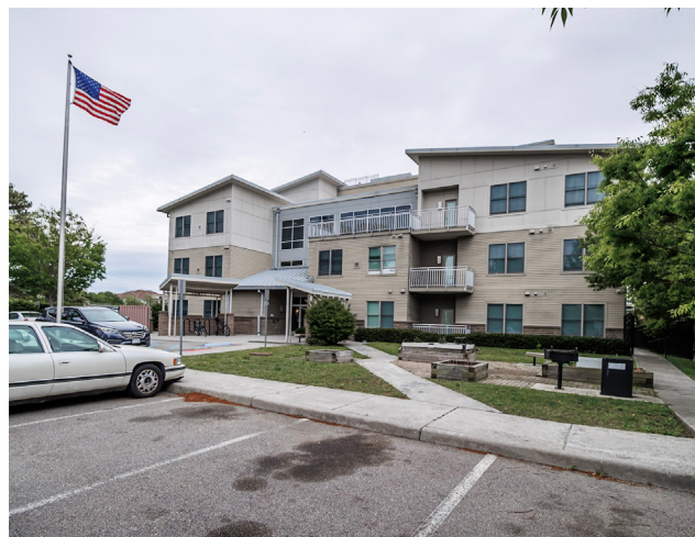
Cedar Grove Apartments
