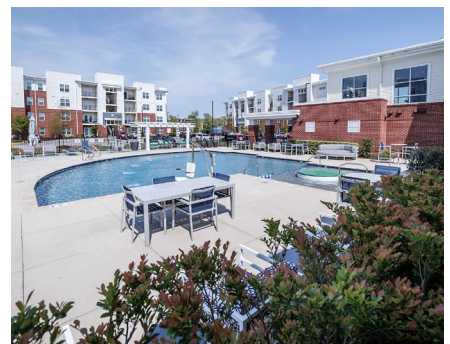
Renaissance Apartments: Mixed-income and serves households with disabilities
