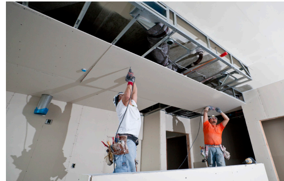
Hanging Drywall on Metal Framework
