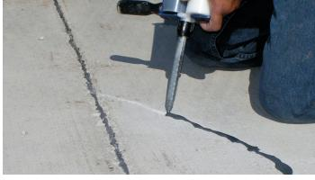
the reinforcement the possibility of corrosion is greatly diminished. The presence of an applied penetrating silane sealer, typical on many deck surfaces, creates a thin hydrophobic protective layer on the surface and provides additional protection against possible corrosion. It should be noted that reapplication is required periodically and manufacturer's recommendations must always be followed.
