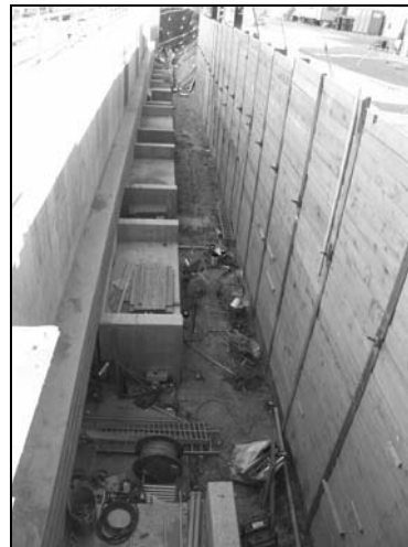
Bill Rodgers/Special to the Daily Press Santa Monica-UCLA Medical Center's new central plant allows the hospital to operate on its own with less energy.
