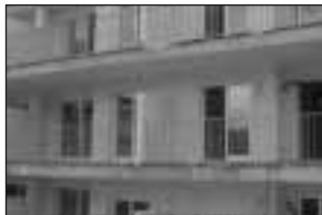
EMPIRE DRIVE 4 UNITS PALMS/MAR VISTA
