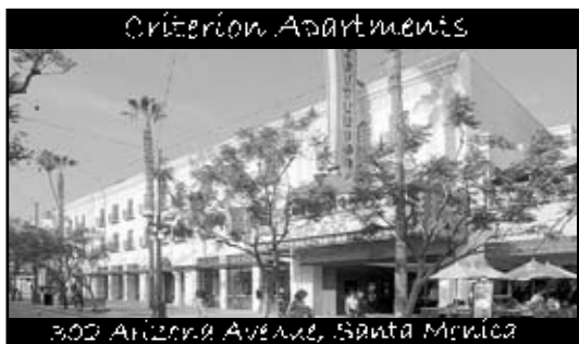
302 Arizona Avenue, Santa Monica
