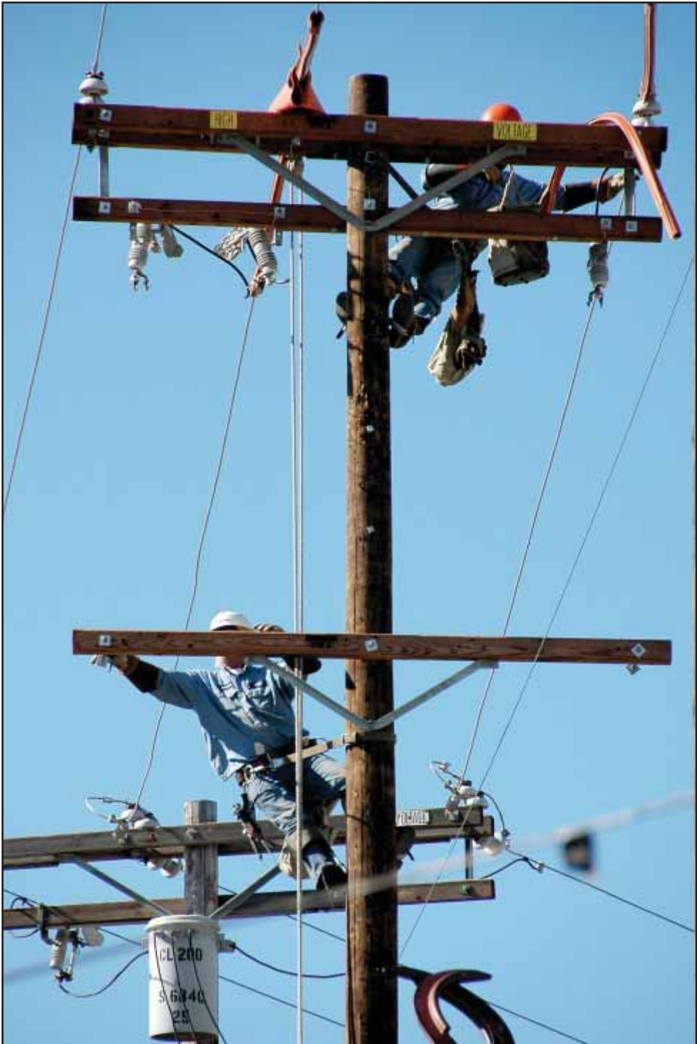
Kinney spirits Fabian Lewkowicz FABIANL@SMDP.COM Chris Sarmiento (at top) and Chuck Berling, from the City of Los Angeles' Water and Power division, work 60 feet up, installing a cross-arm to hold in place a new transformer at the corner of Abbot Kinney and Venice boulevards recently. The extra electricity is needed to build a new development on the lot at corner.
