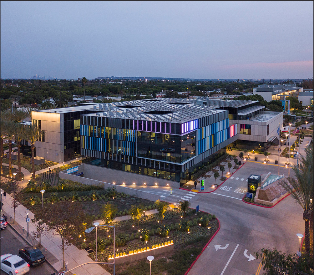
Courtesy Image SMC: Aerial view of Santa Monica College’s Main Campus at 1900 Pico Blvd.
