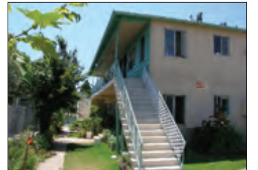
2005 20th St. Santa Monica 6 -1BD/BA Units near Santa Monica College. New Roof $1,048,000
