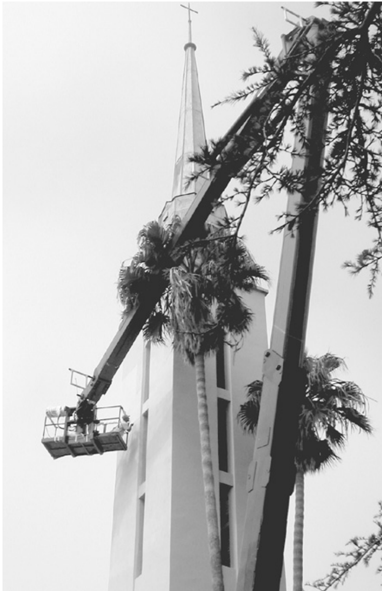
Andrew H. Fixmer/Daily Press The steeple of the First United Methodist Church of Santa Monica on 11th Street and Washington Avenue gets a new coat of paint this week.
