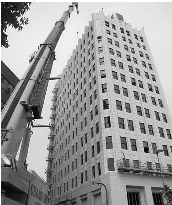
John Wood/Daily Press A crane lifts roofing supplies to the top of the clocktower building in downtown Santa Monica on Thursday. The $60,000 roofing job for the classic building is expected to take two weeks and will begin next week.
