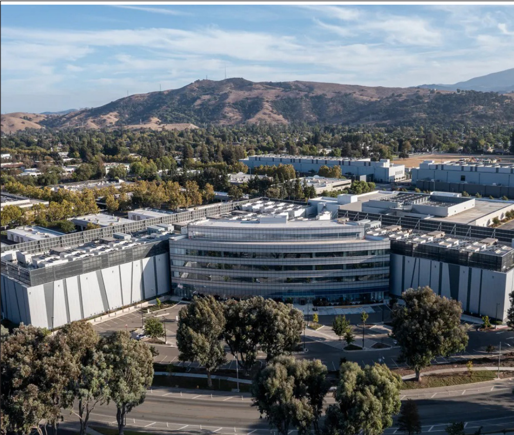
SAN JOSE: A China Mobile data center in South San Jose on Aug. 31, 2026. Photo by Anna Hoch-Kenney, CalMatters
