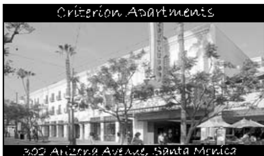
300 Arizona Avenue, Santa Monica
