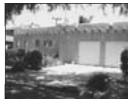
3138 Reid Avenue, Culver City
