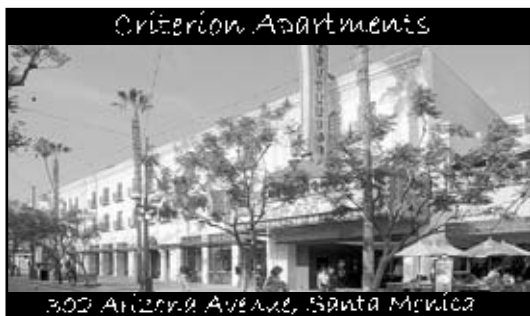
300 Arizona Avenue, Santa Monica
