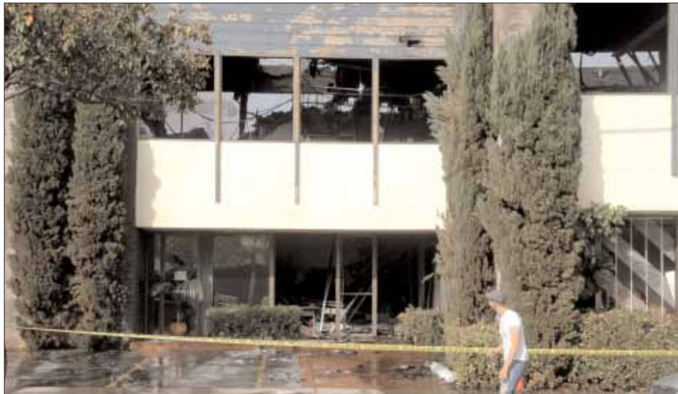
Fabian Lewkowicz fabianl@smdp.com FULLY COOKED: The building at 1928 14th St. was a charred shell following last week's fire.
