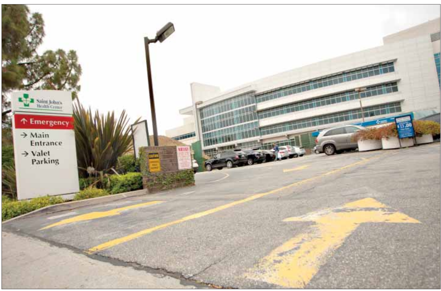
Brandon Wise brandonw@smdp.com NO GO: Saint John's has been absolved by the Planning Commission of building a parking structure. The City Council has final say.
