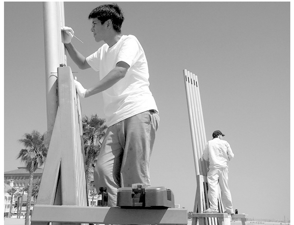
Jeff Chang strips rust from the pipes of a whistling chair on Ocean Front Walk by the Santa Monica Pier this week in preparation for a new coat of paint.
