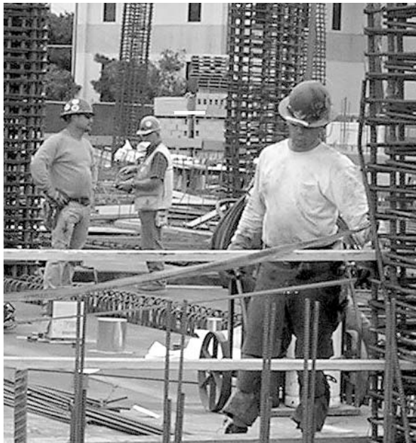
Nicky Five Aces/Special to the Daily Press Workers continue to build the Public Safety Building behind City Hall, which is scheduled to be done by the end of the summer.
