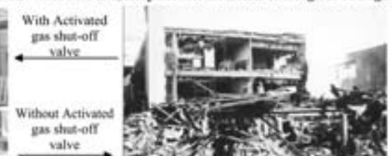
Building demolished due to gas explosion-Lost everything
