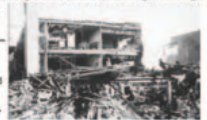
Building demolished due to gas explosion-Lost everything
