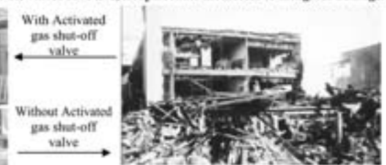
Building demolished due to gas explosion-Lost everything
