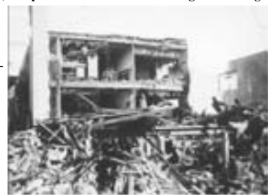
Building demolished due to gas explosion-Lost everything
