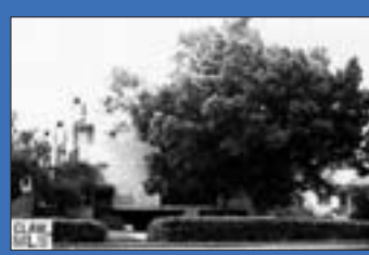
10610 VENICE BLVD. 4 UNITS LOS ANGELES $949,500
