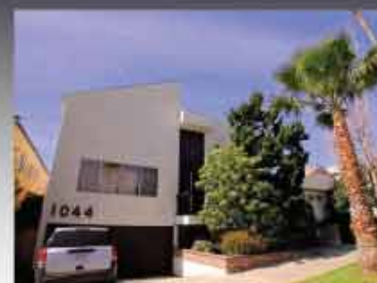
1044 - 19th Street Unit B $794,800 Remodeled 3 + 3.5 Townhome
