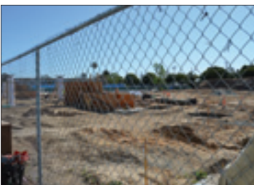
Jeff Goodman jeff@smdp.com ALMOST FINISHED: Work is nearing completion at Edison.
