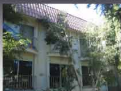
1048 - 9th Street #8 $549,000 Remodeled, Top Floor 1 + 1
