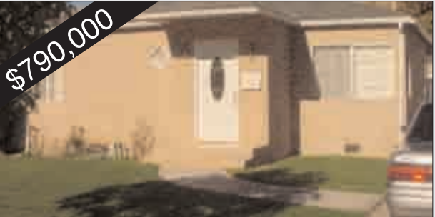
10757 WESTMINSTER AVE. Quiet West LA.neighborhood. Remodeled Kitchen and Bathroom. New Tile Flooring in Kitchen and Bathroom. New Shutters and New Windows. Copper plumbing and upgraded Electrical. Large lot, with great potential for future expansion. Room for swimming pool. According to Seller, the living area is about 1,100sf, with permit. Must see to appreciate.
