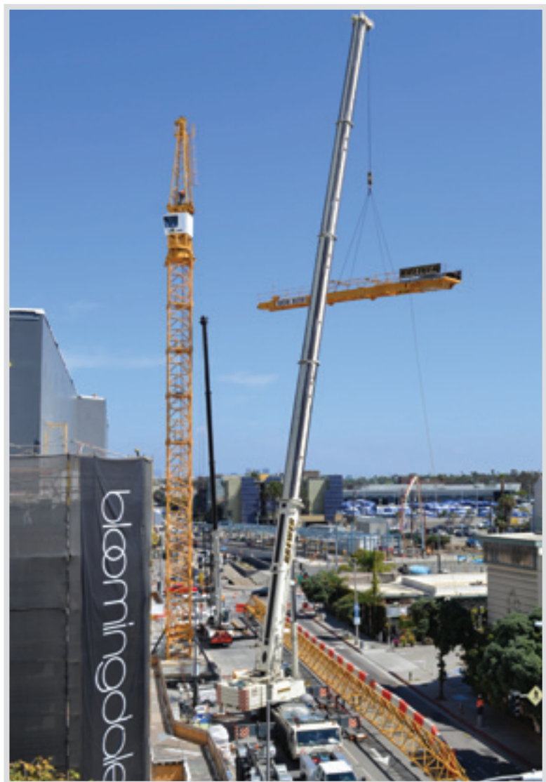
CRANE CAME DOWN Construction crews have removed the large crane from 4th Street that was part of the construction team for the new Arclight movie theater.
