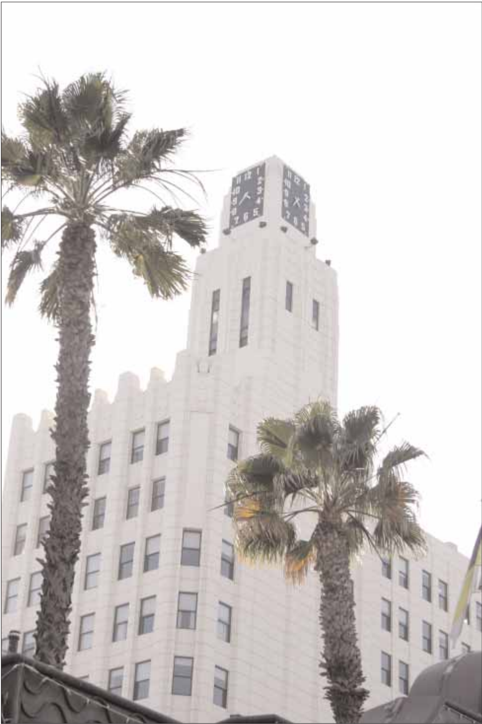
Times are 'a changing The Clock Tower on Santa Monica Boulevard will need to be set early this year.
