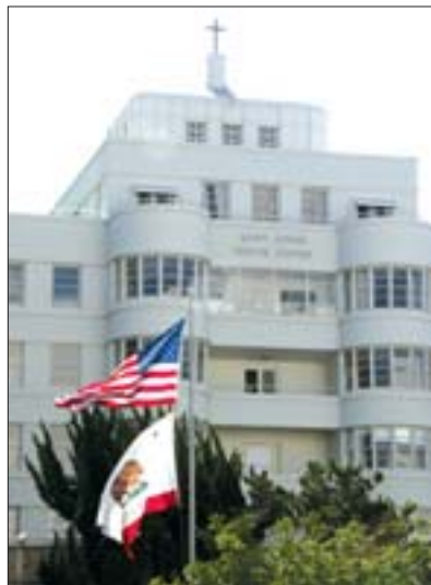
Nicky Five Aces/Five Aces Photography OUT WITH THE OLD: The old Saint John's Healthcare Center building will soon be reduced to rubble.
