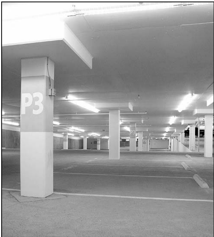
Andrew H. Fixmer/ Daily Press The bottom floor of the city's newest parking garage was completely empty Friday afternoon, though vehicles had filled many of the spaces on the top two floors.
